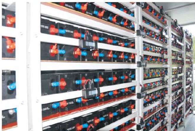
Onsite installation of battery monitoring system
